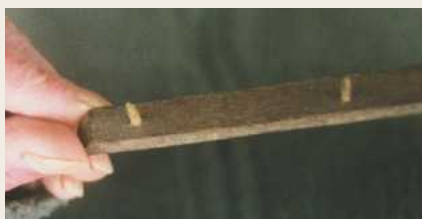
▲ Little things matter: you don’t meet coaks everyday but replace like with like when you do; note the mitre
